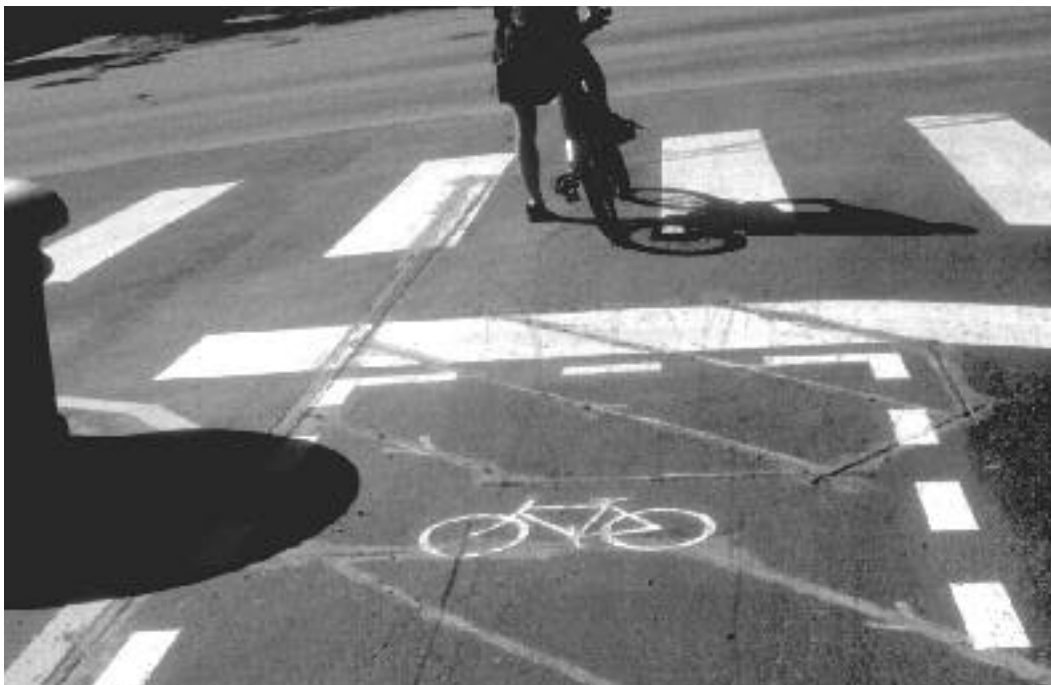
A “Diagonal Quadrupole” traffic signal loop detector that can detect bicycles.
